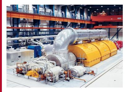
Turbogenerating set of steam turbine (yellow) with synchronous generator (red) *Source: Siemens*
