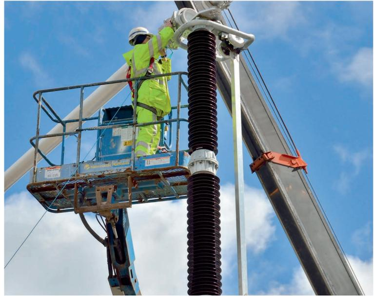
Installing a 400kV Busbar at Moffat Substation
