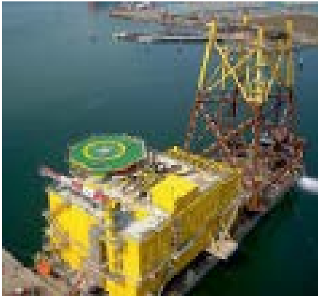
Figure E.17.2 BorWin1 HVDC platform, North Sea. Image courtesy of ABB.
