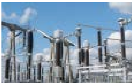
Figure E.4.2 Typical 132kV AIS bay
