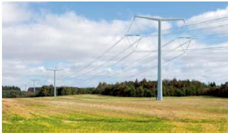
Figure E.1.2 T-pylon
