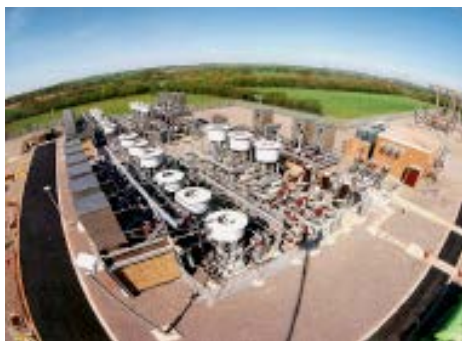
Figure E.8.1 Typical SVC installation
