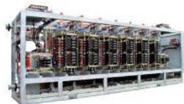
32MVar STATCOM (building required) Image courtesy of ABB
