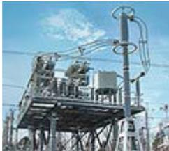
In September 2004 Siemens succeeded in winning the contract for the refurbishment of two series capacitor installations at Edisons Eldorado Substation southwest of Boulder City, Nevada. As a result of new power generation installed in the Las Vegas area the fault duty on the 500 kV transmission network is above the design ratings of the existing equipment and therefore the two series capacitors "Lugo" and "Moenkopi" at the Eldorado Substation were to be replaced.
